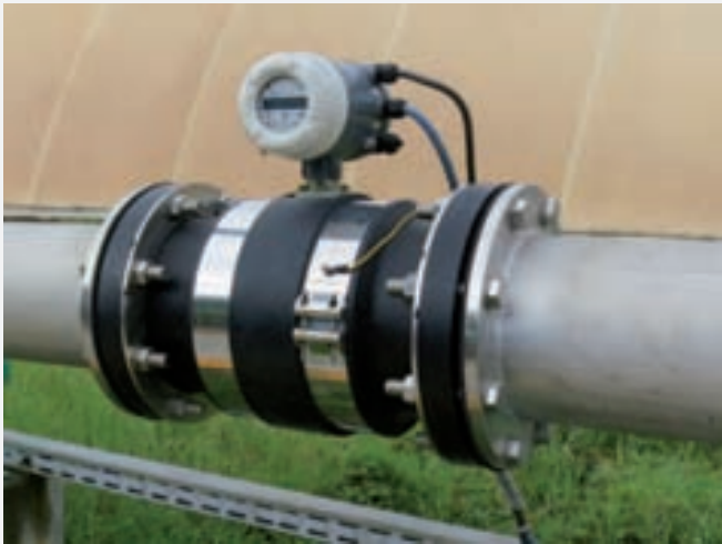
Fig. 5: FLOWSIC600 gas flow meter
