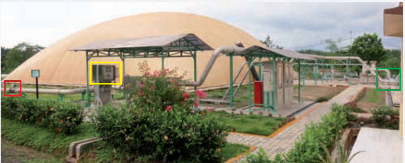
Fig. 1 Belitung plant with gas analyzer (yellow), mass flow meter (red) and gas sampling point (green)
